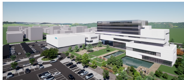
Aerial View of Gwangju National AI Data Center
